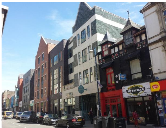
Figure. 5. Urban Village on the Swansea High Street in 2017 [23].
