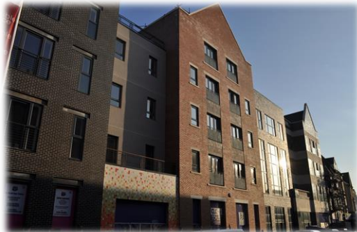
Figure. 4. Urban Village on the Swansea High Street in 2015 [22].
