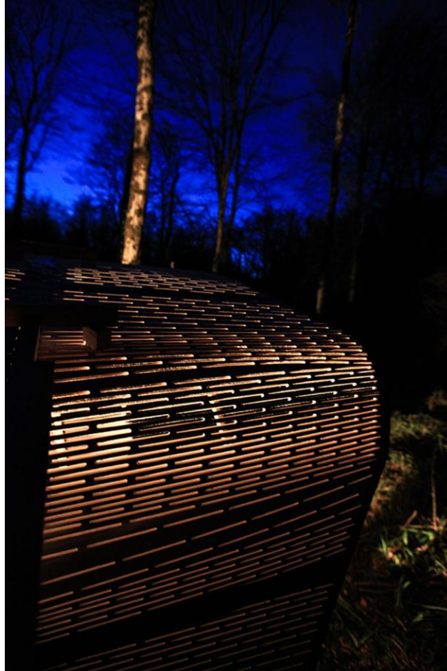
Figure 7. The differentiated slotting pattern on the plywood panels allowed for variable stiffness and emergent lighting effects, although did not provide sufficient structural performance with regard to global stiffness.
